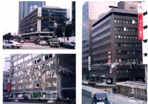
Figure 15 Typical intermediate floor soft-story collapsed buildings during Kobe Earthquake, 1995 (by K. Meguro)
