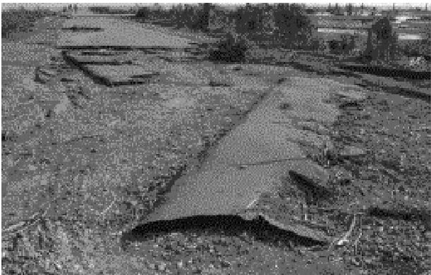
**Figure 4** Coastal Road from Suwak Timah village to Meulaboh. The asphalt also exfoliated and the road surface was damaged in the many areas (left)
