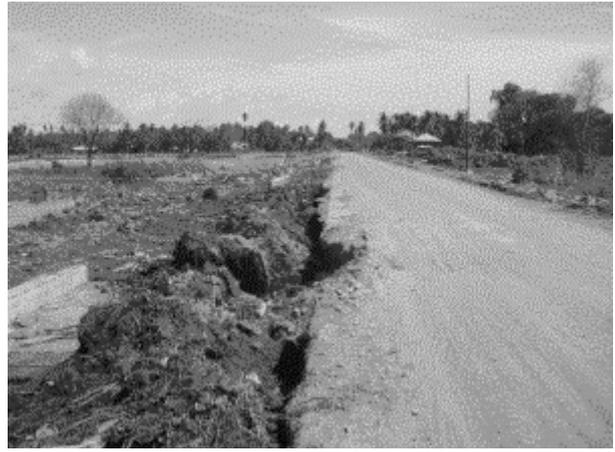
**Figure 3** Road condition near Meulaboh, road shoulder damaged by the tsunamis. (right)
