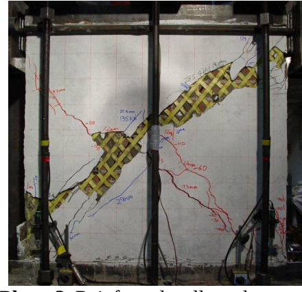
Photo 3. Reinforced wall crack pattern
