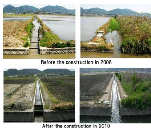
Figure 4 Comparison of irrigation creeks of “before” and “after” the construction in Tsuyazaki. The above pictures show before the construction in 2008, and the pictures below are after the construction in 2010.
