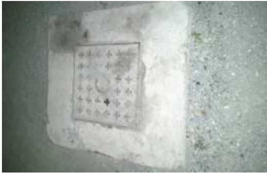
Fig. 6: The PWT Containment System after construction with 546mm diameter Manhole cover.
