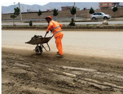
Fig.2 Municipality workers collecting mud after rain.
