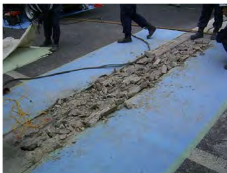
(c) 橋梁の伸縮部取替工事
