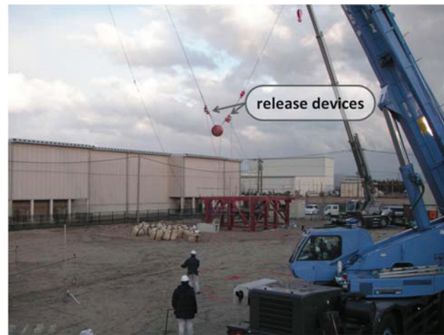
Figure 3: test set up ready to release
