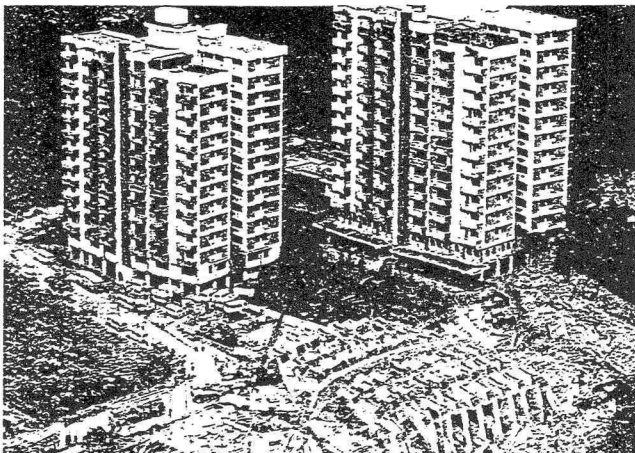
Fig. 2 Air photo of the Highland Towers condominium complex including the collapsed building (Courtesy of New Straight Times , 13 December 1993).
