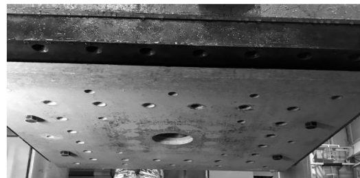
Figure 4. Insulation plate (on the upper surface of specimen)
