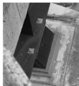
(c) P2 橋脚 G5 支承
