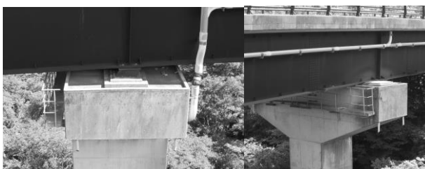
(a) P1橋脚
