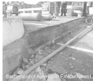
Photo 5 Damage Observation of Tagbuane Br.
