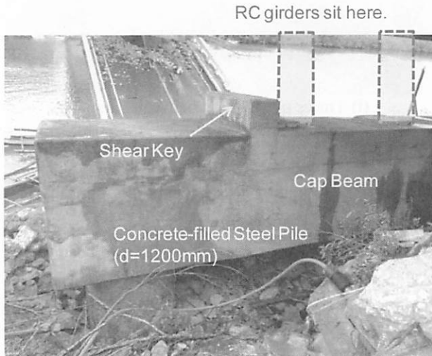
Photo 3 Additional Bent and Shear Key
