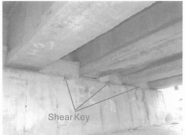
(b) Shear Keys on Seat of Abutment
