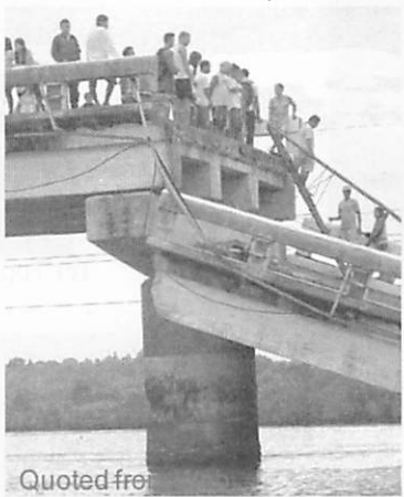
Fig.3 Schematic View of Damage to Abatan Bridge
