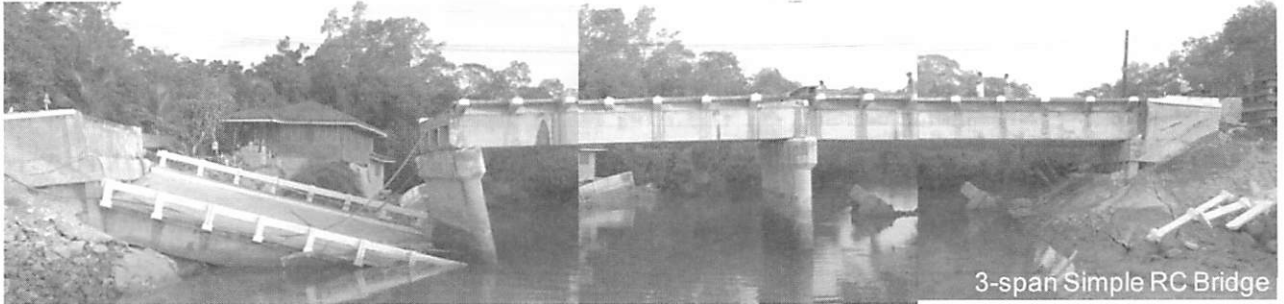
(a) Panoramic View of Moalong Bridge
