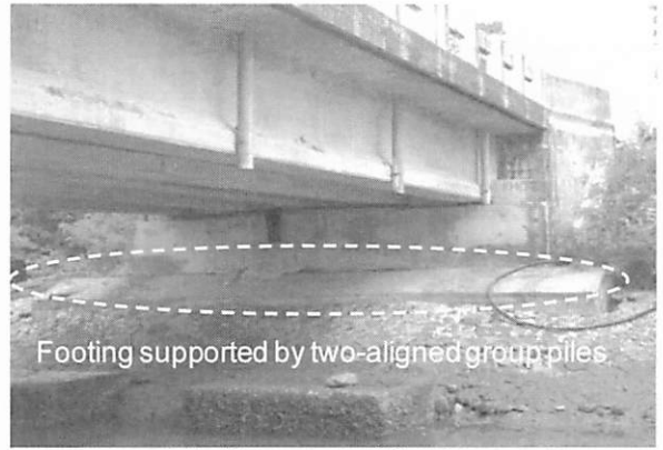
(a) Abutment and Footing
