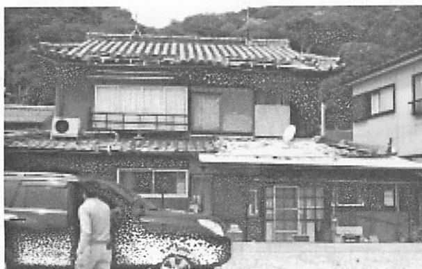
Fig.2 (a) Damages to the roofs and broken tiles of a two storey wooden house at Takenokuchi 2-chome.
