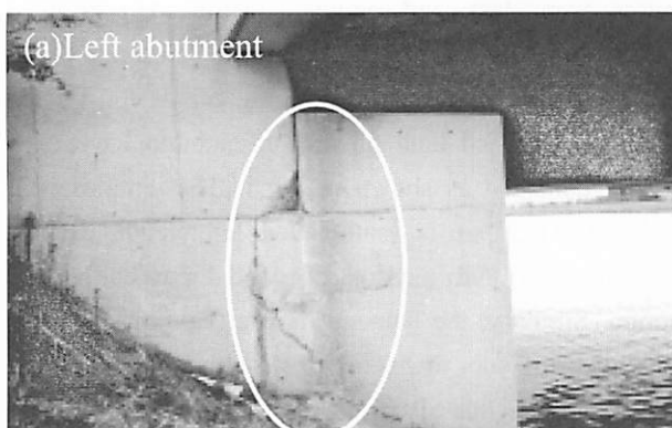
Fig.8 Earthquake damages to the abutments of Suhama Bridge; (a) Cracks on the left abutment; (b) Cracks on the right abutment.
