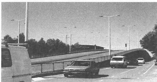
写真-1 Moorhouse Ave/Columbo St 跨道橋の遠景
