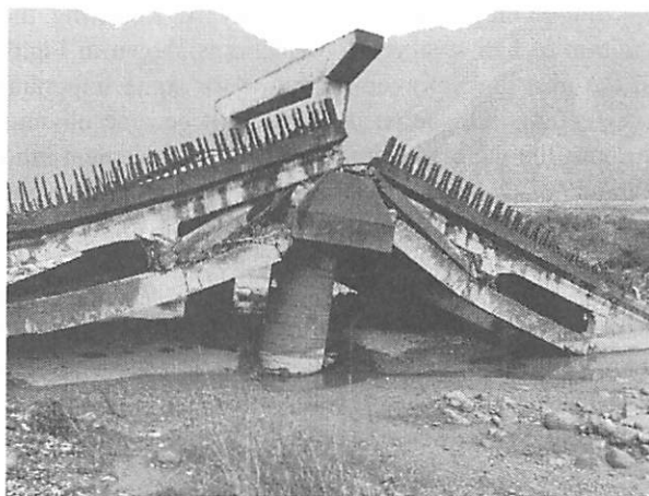
Photo.2 Tilt of Pier 3 (from upstream)
