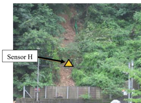
Figure 2: Slope failure in sensor H, Tateyama site
