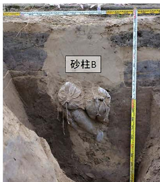
写真-7 B 箇所開削状況
