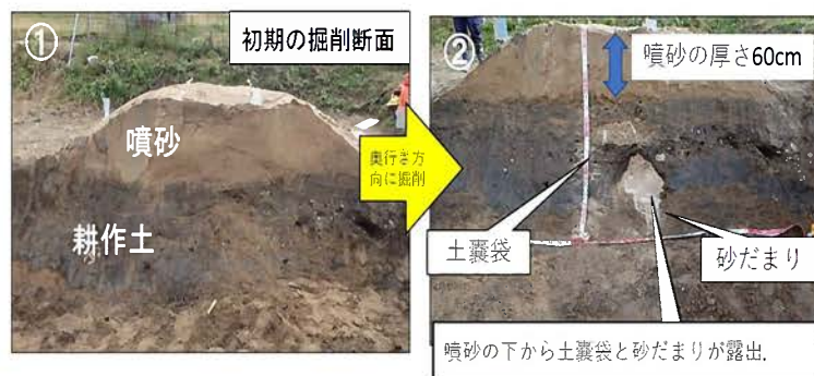
写真-5 A 箇所開削状況
