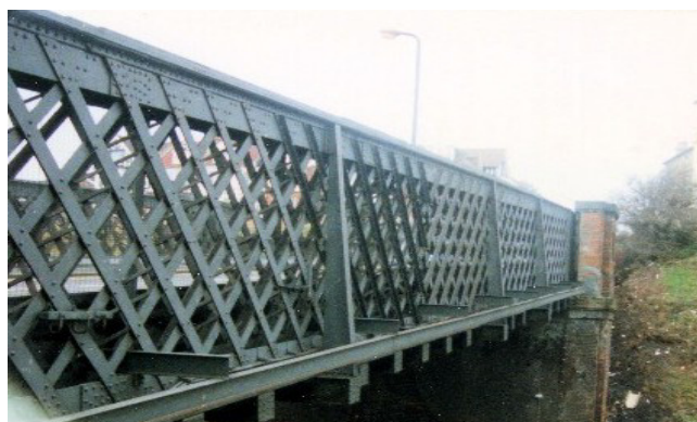
写真-1 Lattice truss
