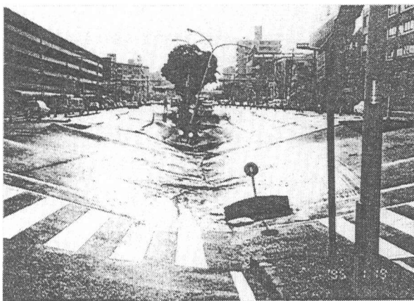
Photo 3 Cave-ins due to the Great Hanshin-Awaji earthquake in January, 1995.
