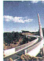
図-2.43 Bridge of R
