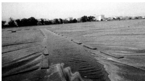
Picture 1. Lagoon covered with black sheet.
