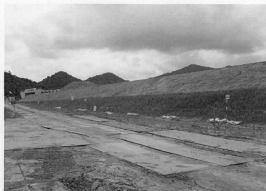
Figure 3 Road construction using excavated rocks
