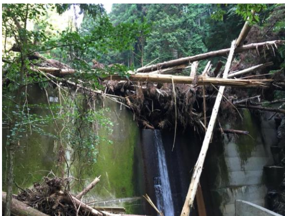
Fig.5. Woody debris trapped at the sabo dam
