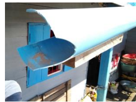
Fig.11 Damaged gutter
