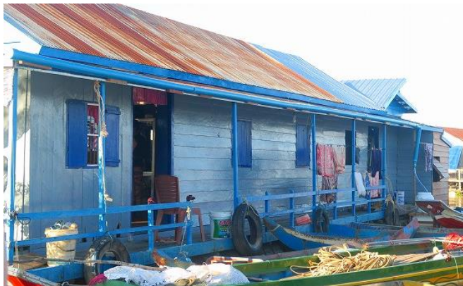
Fig.10 Overall view of rainwater catchment system
