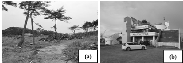
Fig. 3 (a) Damaged control forest in Higashi-Matsushima and (b) Survived evacuation building in Shiogama
