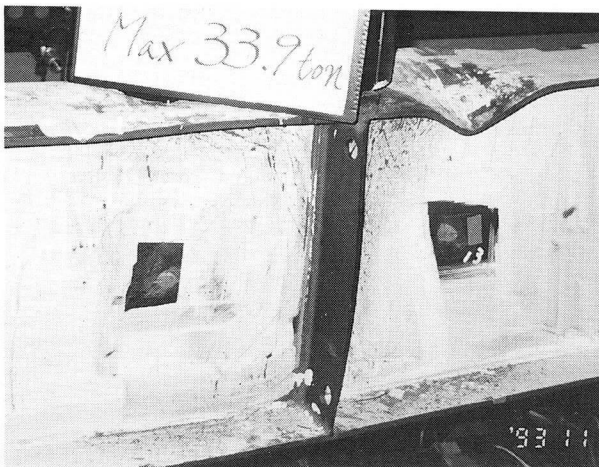
写真-2 Local Buckling of Flanges
