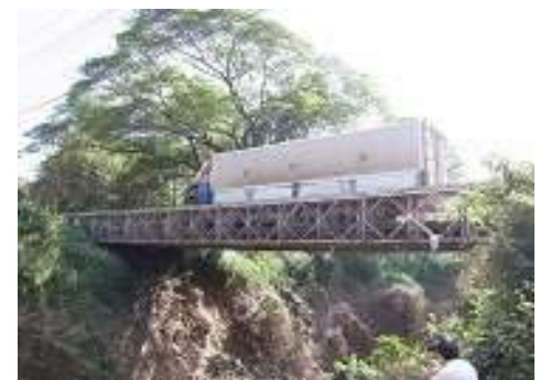
写真 6 Namyong River Bridge
