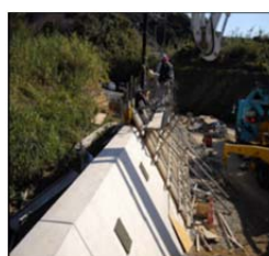
18-8-40BB(Air4.5%) 18-8-40BB(Air3.5%) 18-8-40BB(FA内割20%, Air3.5%) 18-8-40BB(FA外割10%, Air3.5%) 施工日:2009年10月
