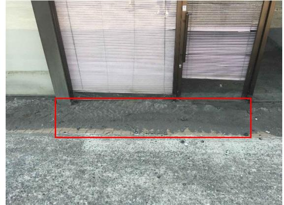
Fig.1 Sand boil of Kumamoto earthquake
