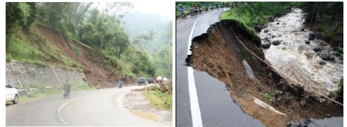
Figure 2. Landslide and slope erosion in the Pujon-Ngantang Road
