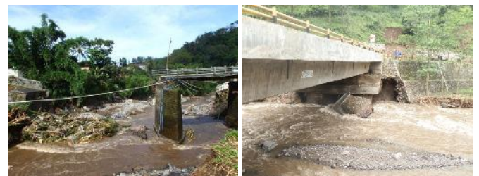
Figure 3. Bridge collapse and damage by flood in the Konto Hulu River
