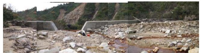
Fig.3. Sediment deposition caused by the upstream check dam of the successive ones (View from upstream to downstream direction on November27, 2009)
