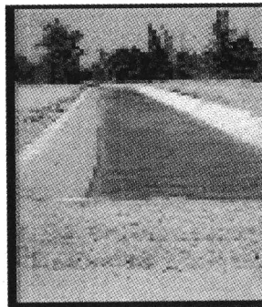
Fig.2 Concrete lining for canals
