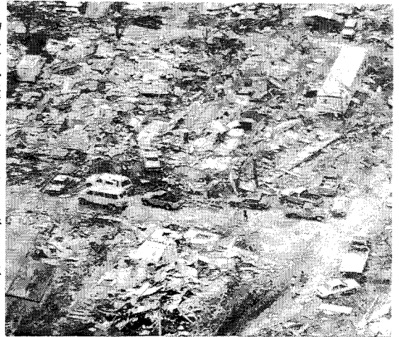
Photo.1 Damage due to Hurricane Andrew
