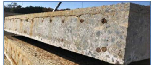
Figure 1 RC bridge deck with SFRC overlay
