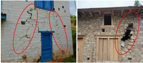
Fig. 4 Diagonal cracks at door and windows opening.
