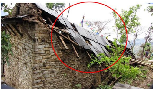
Fig. 5 Roof collapse after damage in support wall
