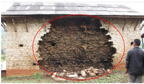
Fig. 3 Collapse of middle portion of long walls.
