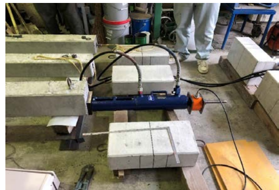
Fig. 2 Installation of hydraulic jack
