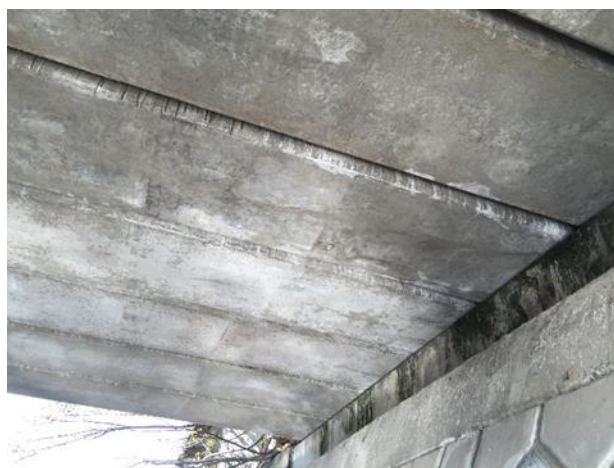
写真-2 橋梁の裏側
