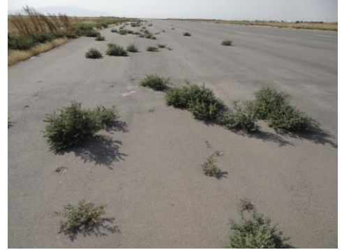
Photo 3. Low Compaction of Runway in Kunduz Airport
