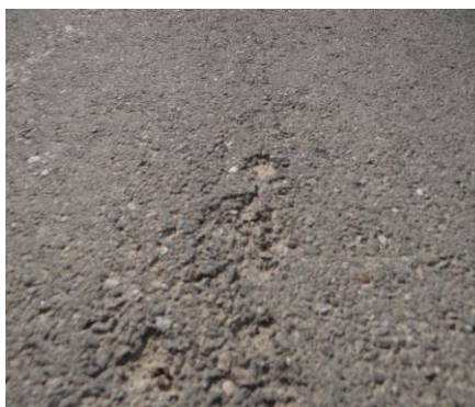
Photo 5. Surface Fatigue of Runway in Kunduz Airport
