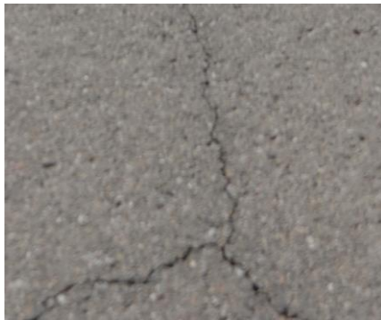
Photo 2. Cracking of Apron in Kabul International Airport
