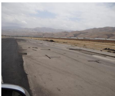
Photo 7, 8,9. Cracking of Runway in Faizabad Airport
