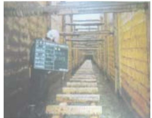
写真-1 はしご胴木基礎<sup>1)</sup>
