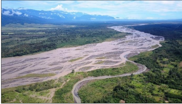
Figure 4. Mavic Pro DJI Drone image of Kesuai Bridge, Ramu Highway, Madang Province, PNG. Photo Credit: Jeremy Mark (2017).
