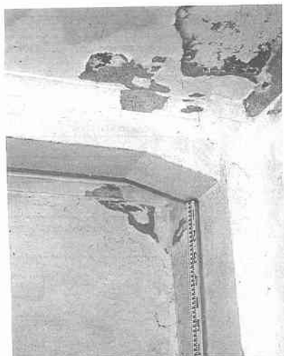
Photo-7 Solid wall girder, ceiling girder and a partition wall between main room and cable-pit room at the center of the interior comparatively one-storied building, as measure for earthquake proofing
