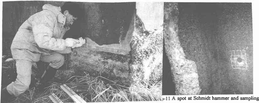
Photo-10 Schmidt hammer test on face of external wall
