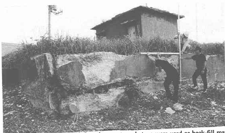
Photo-9 Coastal revetment is reinforced concrete and stone were used as back-fill material.
