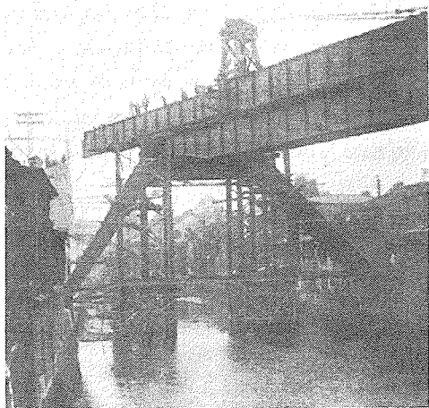
Photo 2 Kandagawa River Bridge (Rigid frame structure, 1932)
