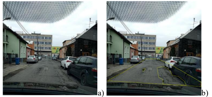
Fig. 10. Road damage image before (a) and after (b) annotation.
