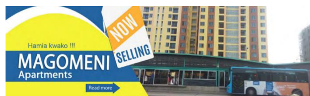
Fig 19: Residential development by WHC alongside the BRT
