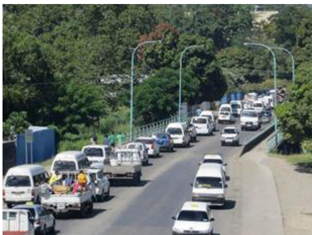
Photo 2.2 New Matanico Bridge
