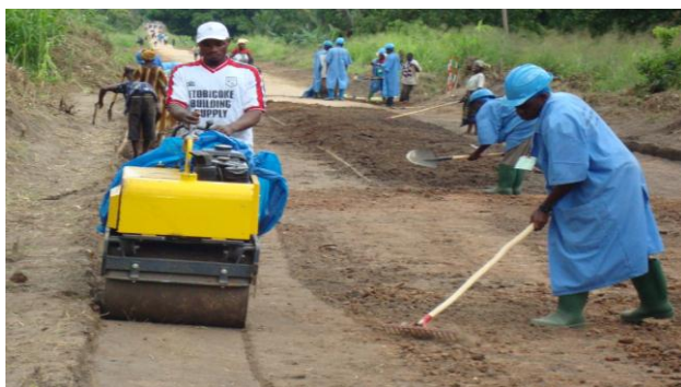
Figure 1 Labour-based road construction works.
