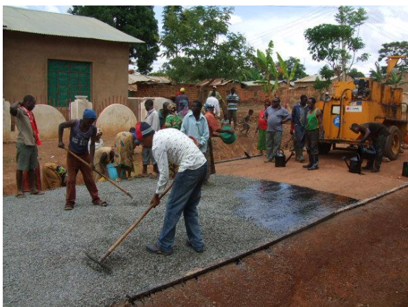
Figure 7 Leveling of aggregates on the prime coat.
