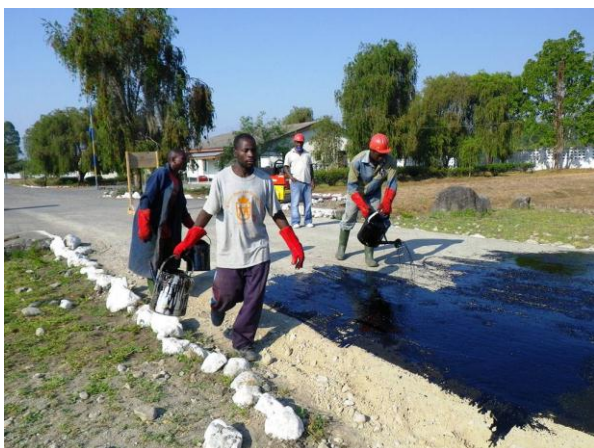
Figure 8 Bitumen brought with a bucket.
