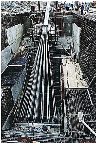
Fig.5 Superstructure Anchorage cable fixing work
