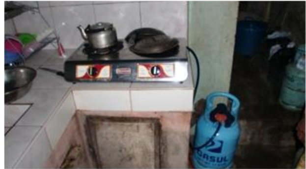
Fig. 17 typical 2-burner LPG stove
