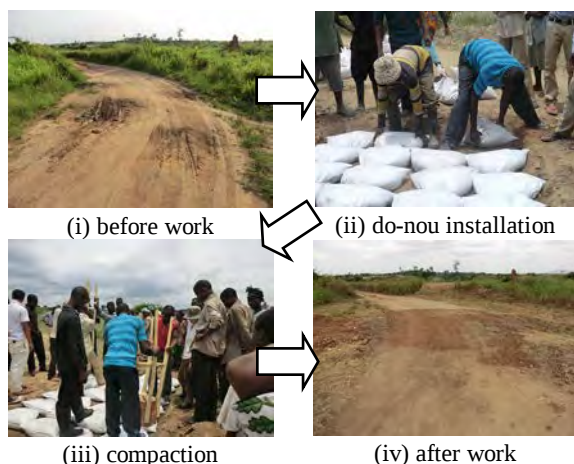
Fig.1 Construction work of the do-nou method (Ghana)
